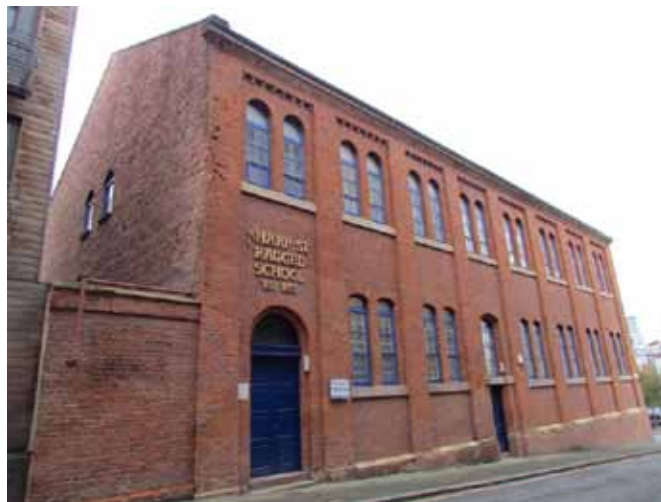
Sharp Street Ragged School, established 1853, now converted into offices Rory Walsh © RGS-IBG Discovering Britain
